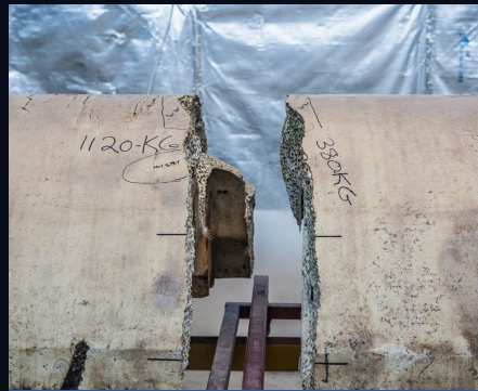
01 Transverse crack repair
