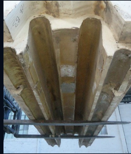
03 Main tube and auxiliary line channels
