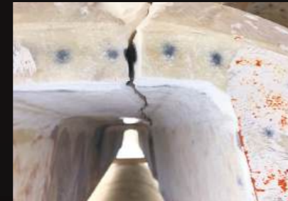
Longitudinal Crack Repair
