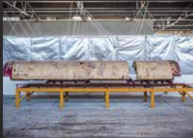
Transverse Crack Repair
