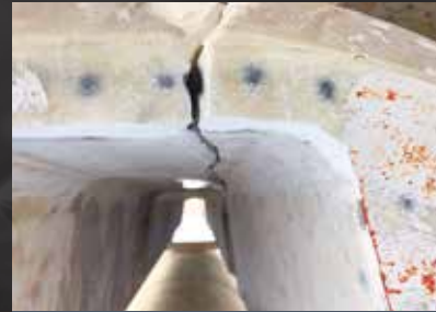
Longitudinal Crack Repair
